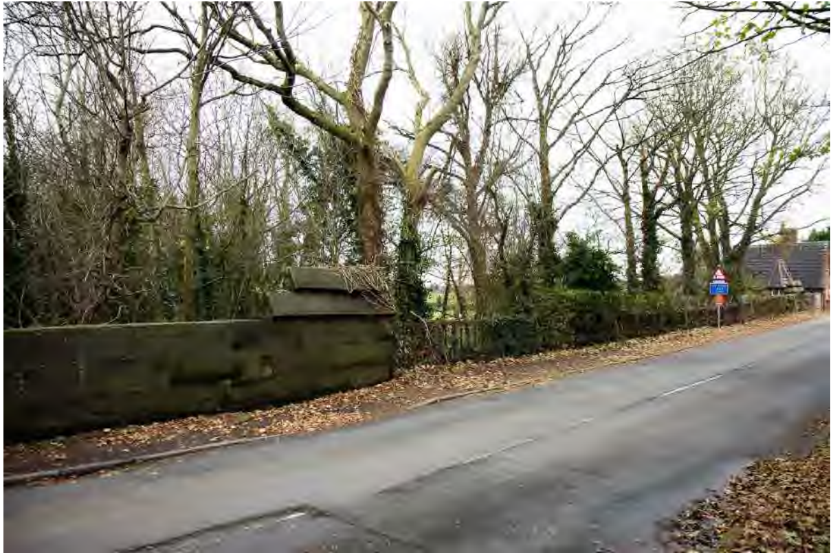
Rixton & Warburton Bridge, November 2021
